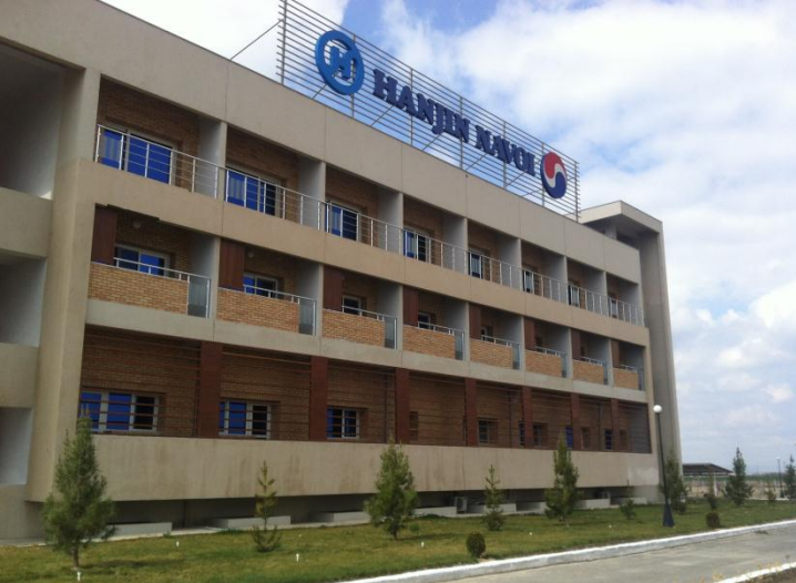
View of B block
