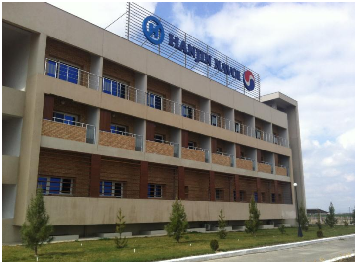
View of B block
